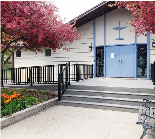
4/22/21 – Completed deck, steps and handicap ramp with metal railings at the church entrance. A center railing will be installed.
