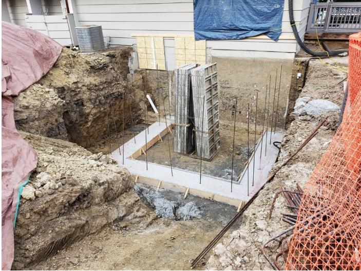
June 30-Basement footings have been poured.
