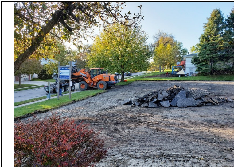
Demolition of the old asphalt parking lot Oct. 22, 2019
