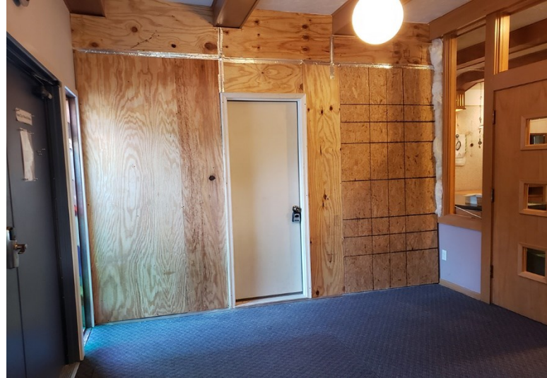
Temporary wall on west side of Church Entryway.
